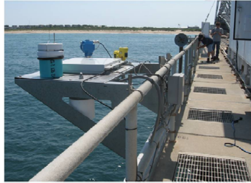
Figure 5. Sensors in mounting plate attached to pier railing at the Duck, NC field test site.
